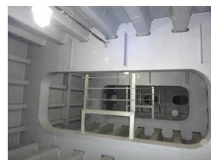
Figure 2. The internal steel box girder
